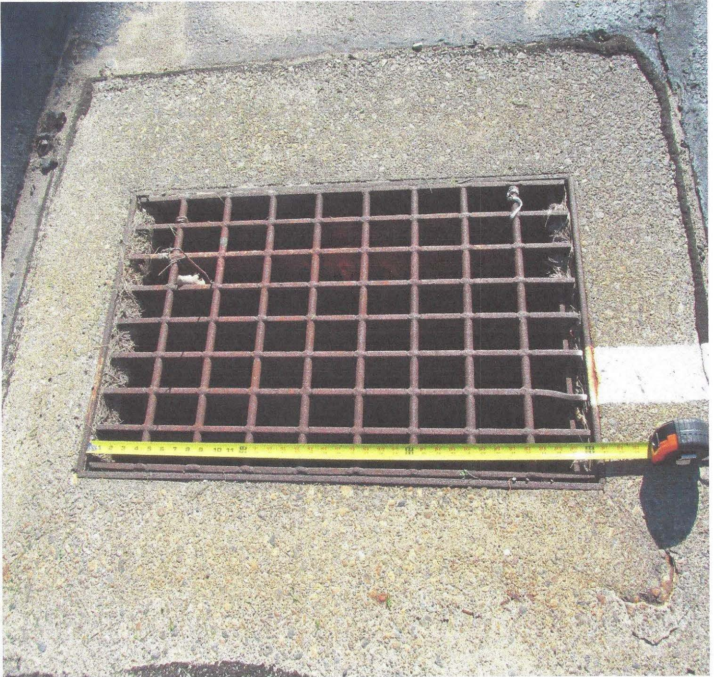
Storm Drain 18" x 36" Metal Grate located 29 Feet From Proposed Propane Dispenser/Refill Station
