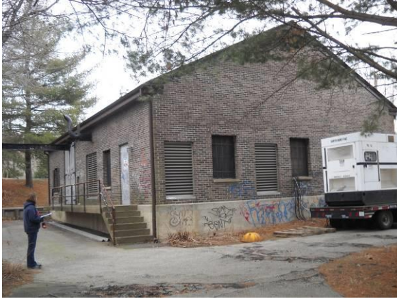
Beardsley Pump Station - West Wall
