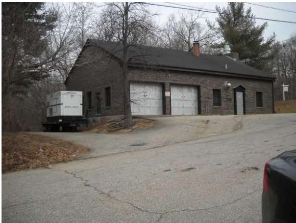
Beardsley Pump Station - Front View
