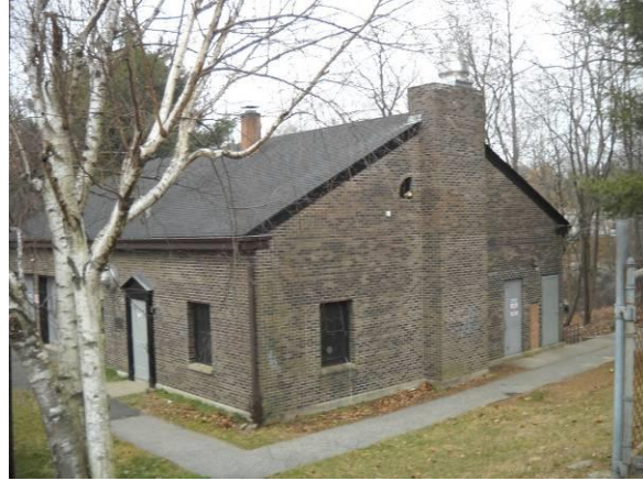
Beardsley Pump Station - East Wall
