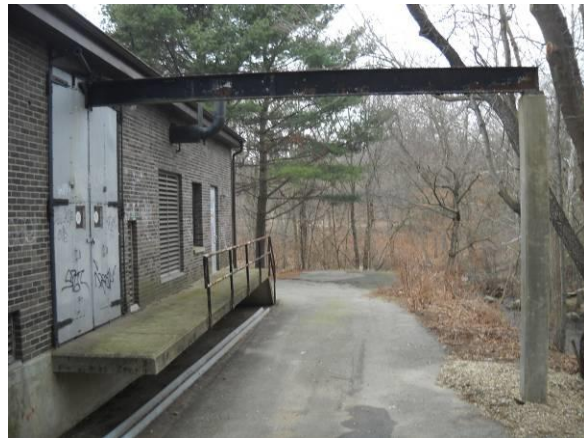
Beardsley Pump Station - Rear View
