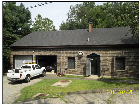
Beardsley Pump Station
