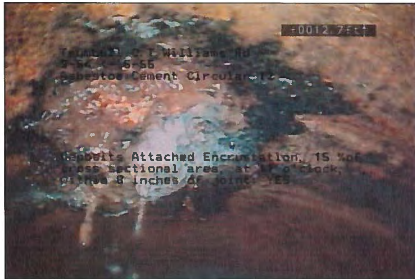
Photo: 220_221_1222_A.JPG, VCR No.: disc #21 12.7FT, Deposits Attached Encrustation, 15 % of Cross Sectional Area, at 11 o'clock, within 8 inches of joint: YES
