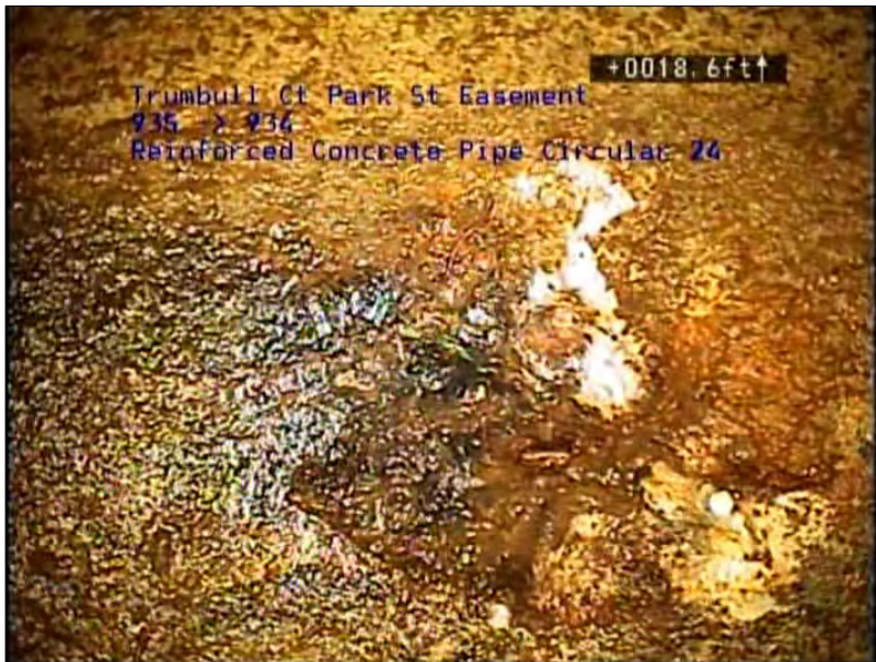
Photo: 483_483_2441_A.jpg, VCR No.: 43 18.6FT, Hole Soil Visible, at 12 o'clock, within 8 inches of joint: NO
