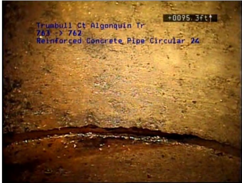
Photo: 516_516_2604_A.jpg, VCR No.: 47 95.4FT, Infiltration Runner, from 06 to 09 o'clock, within 8 inches of joint: YES
