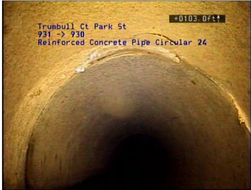
Photo: 499_499_2517_A.jpg, VCR No.: 45 103FT, Broken, from 10 to 12 o'clock, within 8 inches of joint: YES
