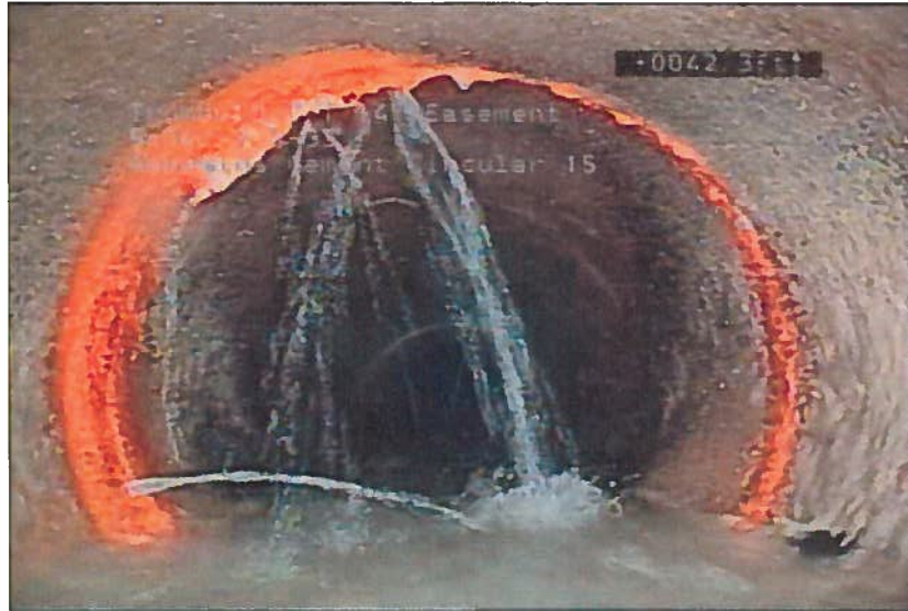
Photo: 154_155_960_A.JPG, VCR No.: disc #17 42.3FT, Infiltration Gusher, from 12 to 12 o'clock, within 8 inches of joint: YES
