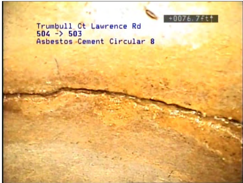
Photo: 241_241_1251_A.jpg, VCR No.: Disc 20 76.7FT, Infiltration Runner, from 12 to 11 o'clock, within 8 inches of joint: NO
