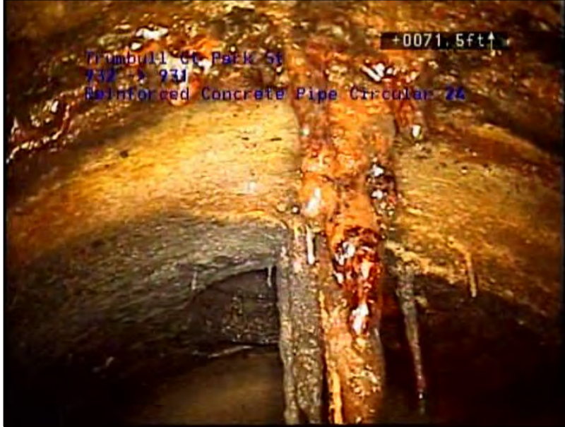
Photo: 498_498_2509_A.jpg, VCR No.: 44 71.5FT, Infiltration Runner, from 06 to 10 o'clock, within 8 inches of joint: YES
