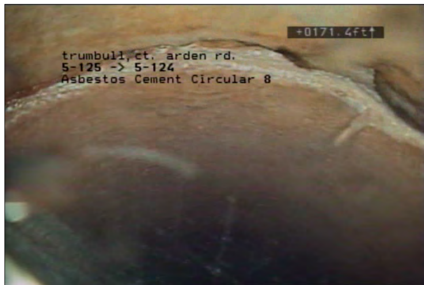
Photo: 375_376_2231_A.jpg, VCR No.: 22 171.7FT, Broken Soil Visible, from 07 to 06 o'clock, within 8 inches of joint: NO
