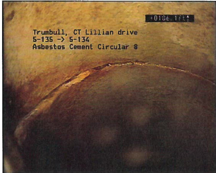
Photo: 17_18_130_A.JPG, VCR No.: Tape 1 186FT, Infiltration Gusher, from 06 to 09 o'clock, within 8 inches of joint: NO
