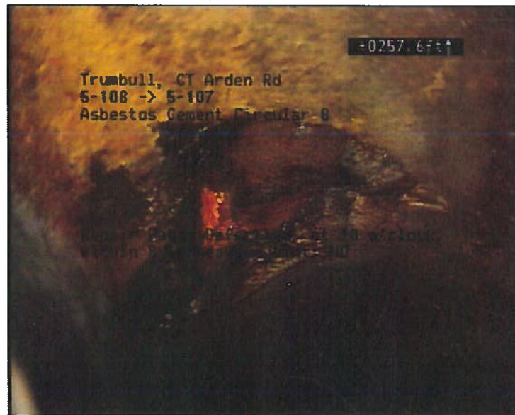
Photo: 31_32_263_A.JPG, VCR No.: Tape 1 257.6FT, Repair Patch Defective, at 10 o'clock, within 8 inches of joint: NO
