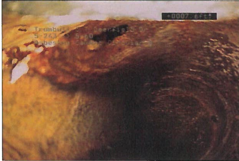
Photo: 114_115_739_A.JPG, VCR No.: disc #13 7.6FT, Tap Factory Made Defective, at 10 o'clock, 6", within 8 inches of joint: NO
