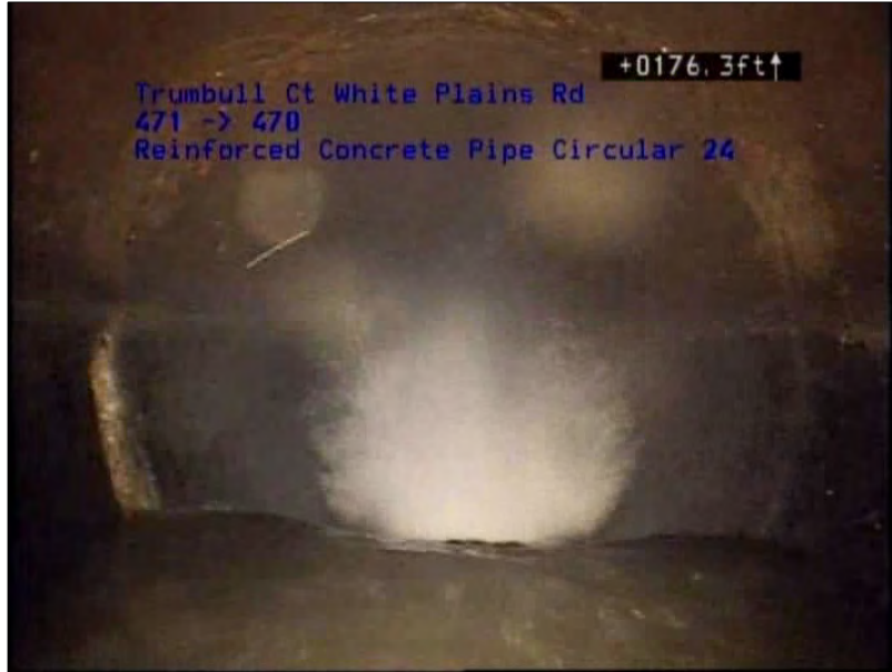
Photo: 524_524_2632_A.jpg, VCR No.: 47 176.3FT, Infiltration Gusher, at 10 o'clock, within 8 inches of joint: YES
