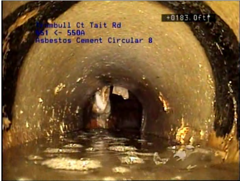
Photo: 334_334_1689_A.jpg, VCR No.: Disc 28 183.4FT, Infiltration Gusher, at 04 o'clock, within 8 inches of joint: YES
