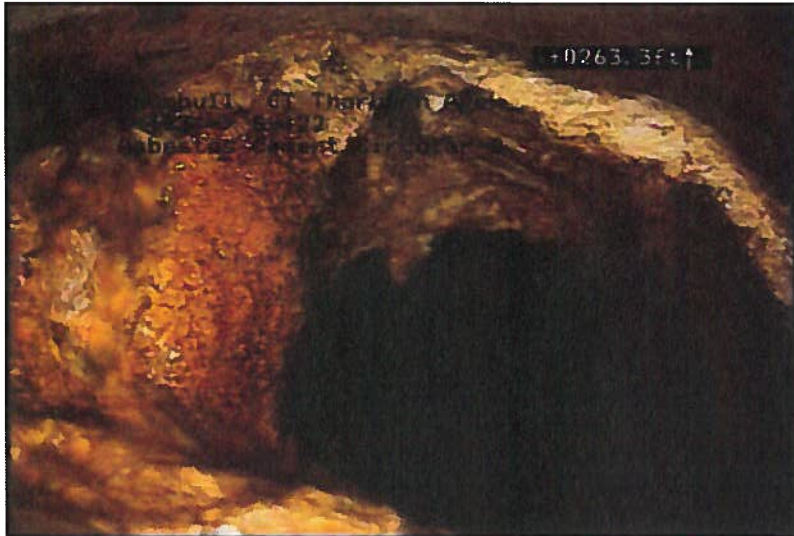
Photo: 10_11_79_A.jpg, VCR No.: Tape 1 263.6FT, Infiltration Gusher, at 10 o'clock, within 8 inches of joint: NO
