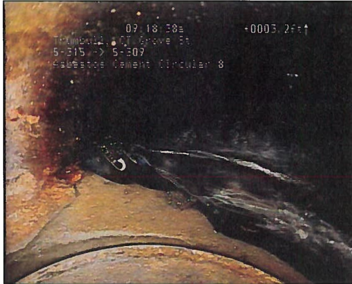
Photo: 73_74_520_A.JPG, VCR No.: Tape #4 3.2FT, Infiltration Gusher, at 02 o'clock, within 8 inches of joint: YES
