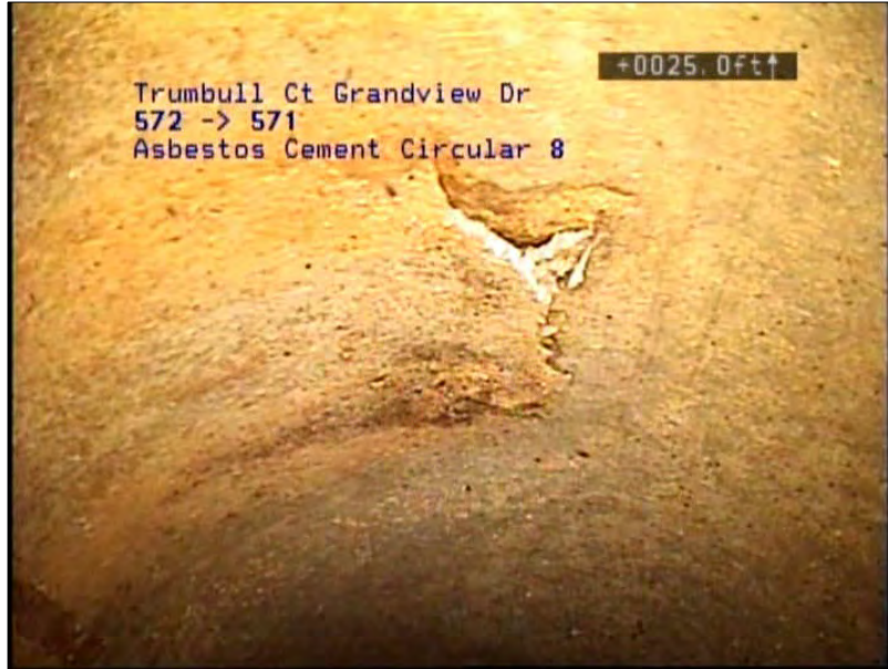
Photo: 252_252_1324_A.jpg, VCR No.: Disc 22 25FT, Broken, from 09 to 10 o'clock, within 8 inches of joint: NO
