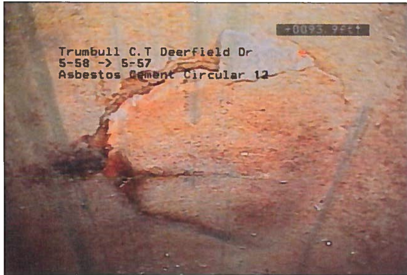
Photo: 232_233_1281_A.JPG, VCR No.: disc #22 93.9FT, Broken, at 12 o'clock, within 8 inches of joint: NO
