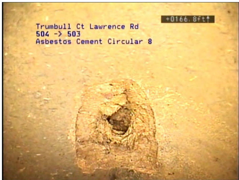
Photo: 241_241_1253_A.jpg, VCR No.: Disc 20 166.8FT, Hole Void Visible, at 01 o'clock, within 8 inches of joint: NO
