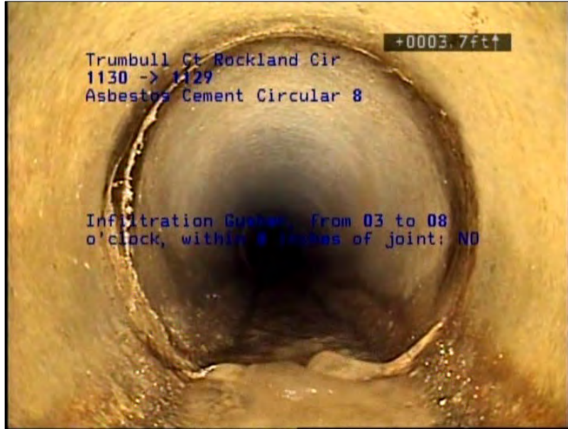
Photo: 302_302_1542_A.jpg, VCR No.: Disc 26 3.7FT, Infiltration Gusher, from 03 to 08 o'clock, within 8 inches of joint: NO NO
