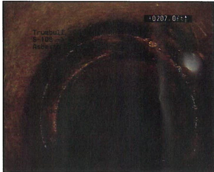
Photo: 31_32_262_A.JPG, VCR No.: Tape 1 207FT, Deposits Attached Encrustation, 5 % of Cross Sectional Area, From 12 to 12 o'clock, Within 8 inches of joint: YES
