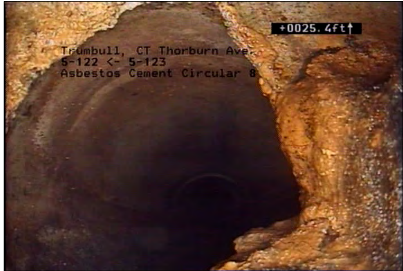
Photo: 11_12_86_A.jpg, VCR No.: Tape 1 25.4FT, Deposits Attached Encrustation, 30 % of Cross Sectional Area, At 02 o'clock, Within 8 inches of joint: NO
