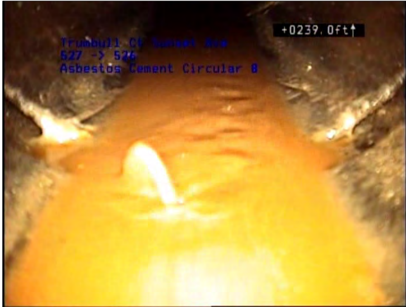
Photo: 281_281_1459_A.jpg, VCR No.: Disc 24 239FT, Infiltration Gusher, at 06 o'clock, within 8 inches of joint: YES
