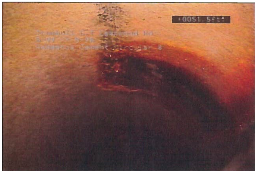
Photo: 46_47_273_A.JPG, VCR No.: disc #6 51.5FT, Infiltration Weeper, at 02 o'clock, within 8 inches of joint: NO
