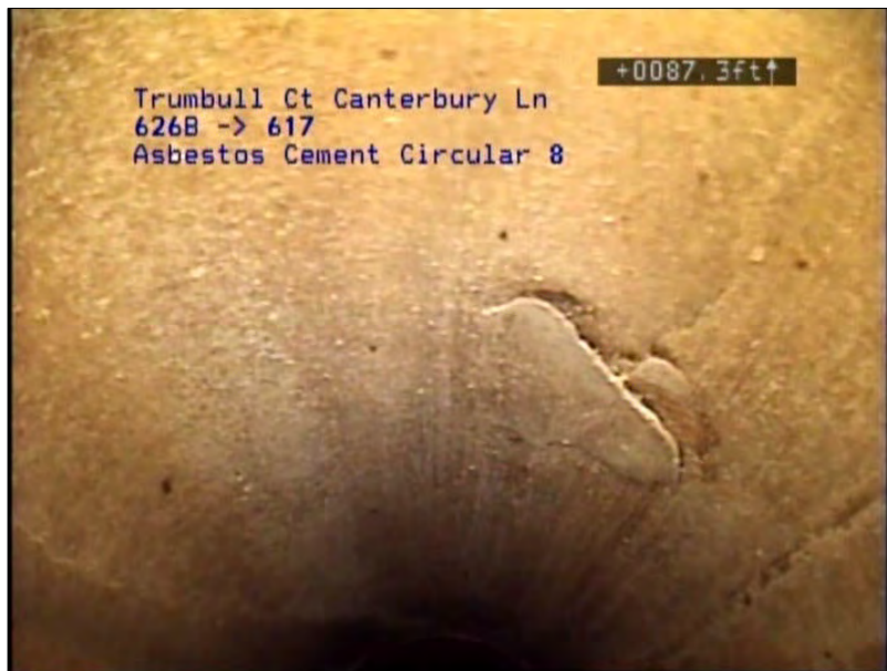
Photo: 155_155_857_A.jpg, VCR No.: Disc 12 87.3FT, Broken, from 12 to 01 o'clock, within 8 inches of joint: NO
