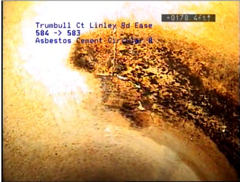
Photo: 187_187_979_A.jpg, VCR No.: Disc 15 178.4FT, Broken, from 01 to 02 o'clock, within 8 inches of joint: NO
