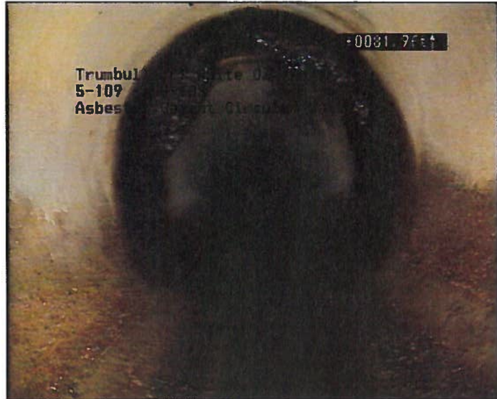
Photo: 30_31_252_A.JPG, VCR No.: Tape 1 81.9FT, Deposits Attached Encrustation, 10 % of Cross Sectional Area, From 12 to 11 o'clock, Within 8 inches of joint: YES
