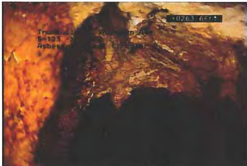
Photo: 10_11_80_A.jpg, VCR No.: Tape 1 263.6FT, Deposits Attached Encrustation, 30 % of Cross Sectional Area, at 10 o'clock, Within 8 inches of joint: NO
