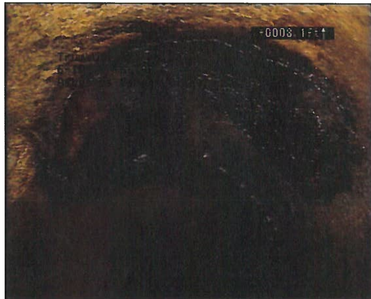
Photo: 30_31_250_A.JPG, VCR No.: Tape 1 8.1FT, Deposits Attached Encrustation, 5 % of Cross Sectional Area, From 12 to 04 o'clock, Within 8 inches of joint: NO
