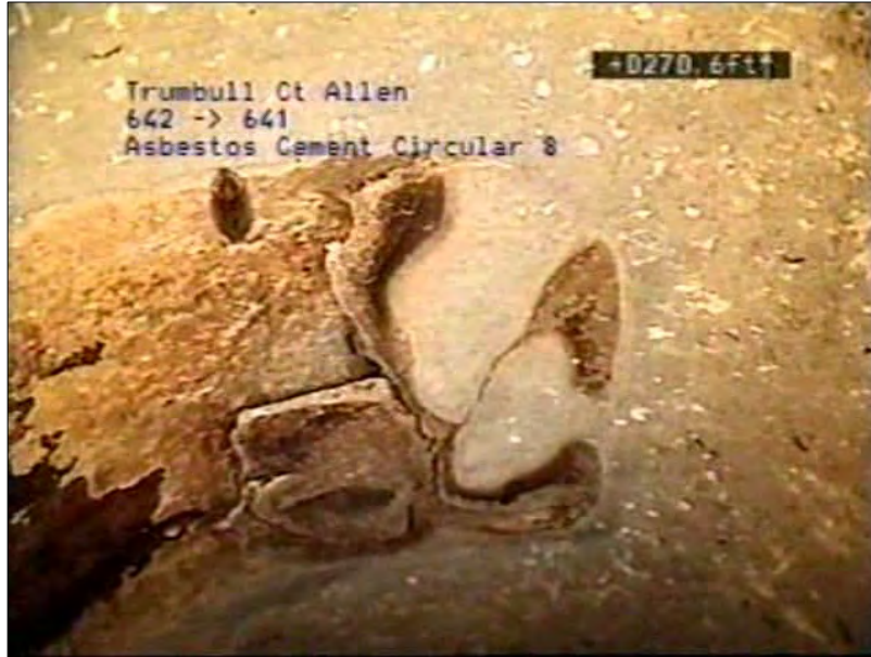
Photo: 56_56_328_A.jpg, VCR No.: Disc 7 270.6FT, Broken, at 11 o'clock, within 8 inches of joint: NO
