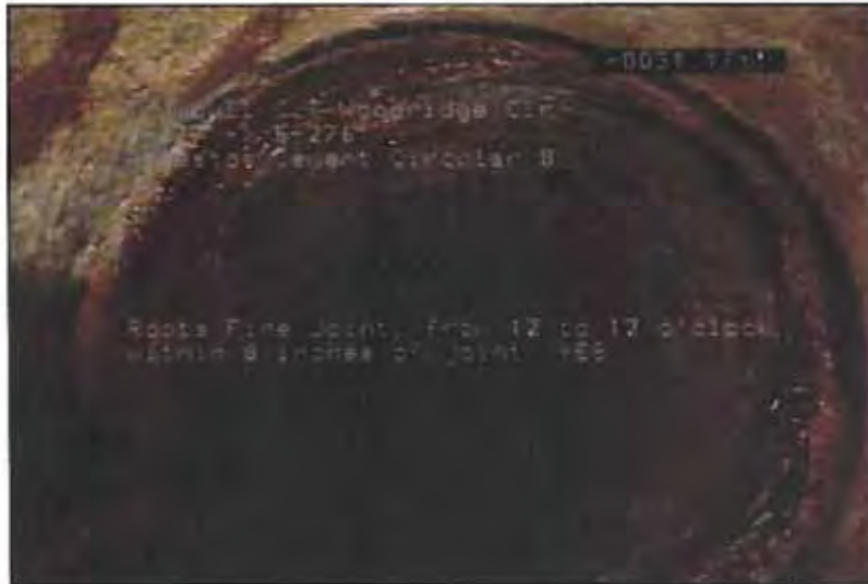
Photo: 84_85_541_A.JPG, VCR No.: disc #10 31.1FT, Roots Fine Joint, from 12 to 12 o'clock, within 8 inches of joint: YES
