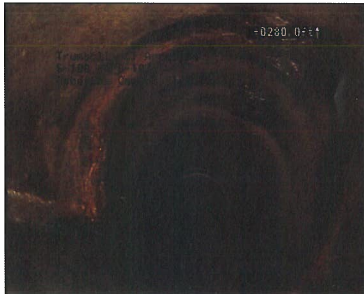
Photo: 31_32_265_A.JPG, VCR No.: Tape 1 280FT, Infiltration Runner, at 10 o'clock, within 8 inches of joint: YES
