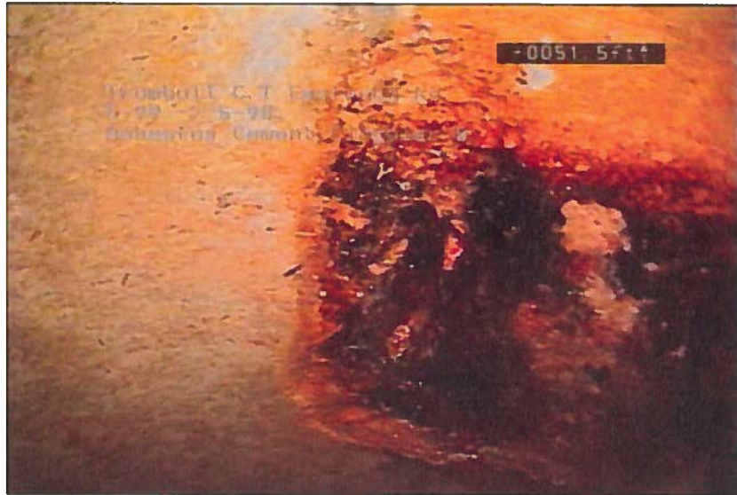
Photo: 46_47_272_A.JPG, VCR No.: disc #6 51.5FT, Hole Void Visible, at 02 o'clock, within 8 inches of joint: NO
