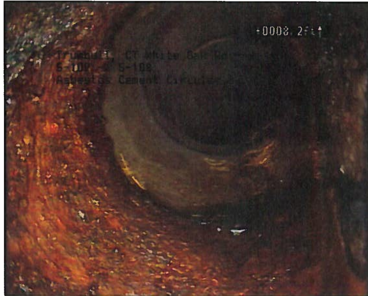
Photo: 30_31_249_A.JPG, VCR No.: Tape 1 8.1FT, Tap Saddle Defective, at 02 o'clock, 6", within 8 inches of joint: NO
