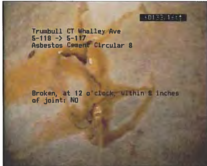
Photo: 1_1_6_A.JPG, VCR No.: Tape 1 133.1FT, Broken, at 12 o'clock, within 8 inches of joint: NO
