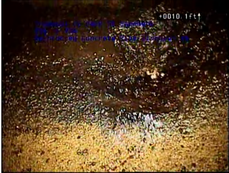
Photo: 483_483_2438_A.jpg, VCR No.: 43 10.3FT, Hole Soil Visible, at 12 o'clock, within 8 inches of joint: YES
