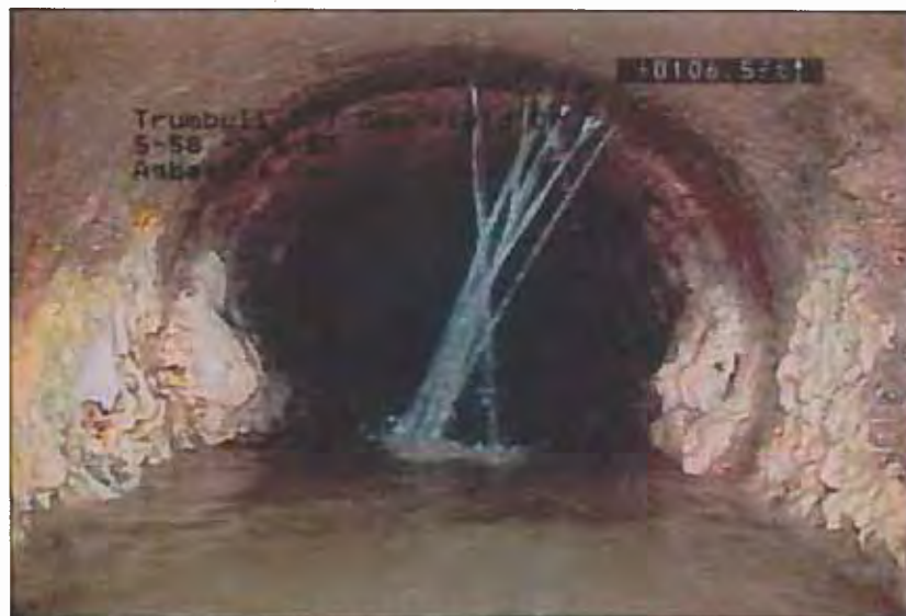
Photo: 232_233_1282_A.JPG, VCR No.: disc #22 106.5FT, Infiltration Gusher, from 12 to 01 o'clock, within 8 inches of joint: YES
