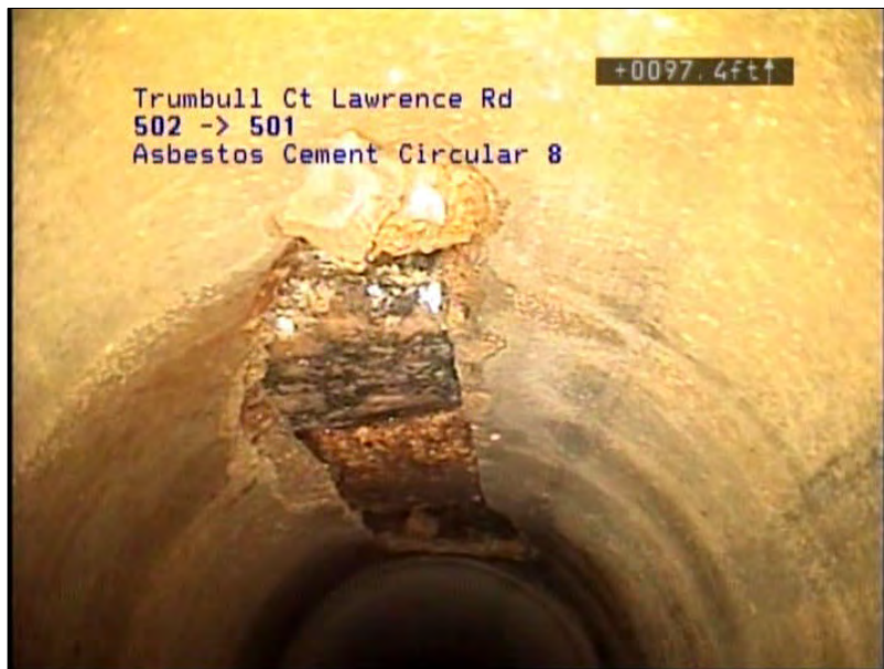
Photo: 245_245_1286_A.jpg, VCR No.: Disc 21 97.4FT, Hole Void Visible, from 11 to 01 o'clock, within 8 inches of joint: YES
