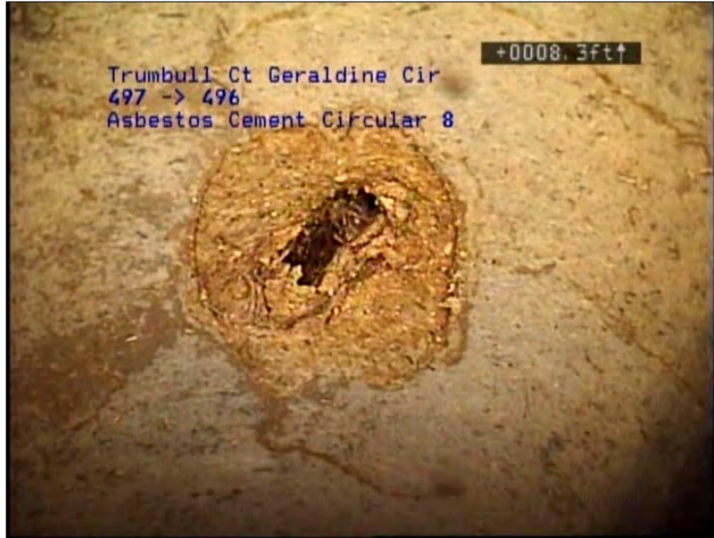
Photo: 213_213_1121_A.jpg, VCR No.: Disc 16 8.3FT, Hole Soil Visible, at 12 o'clock, within 8 inches of joint: NO
