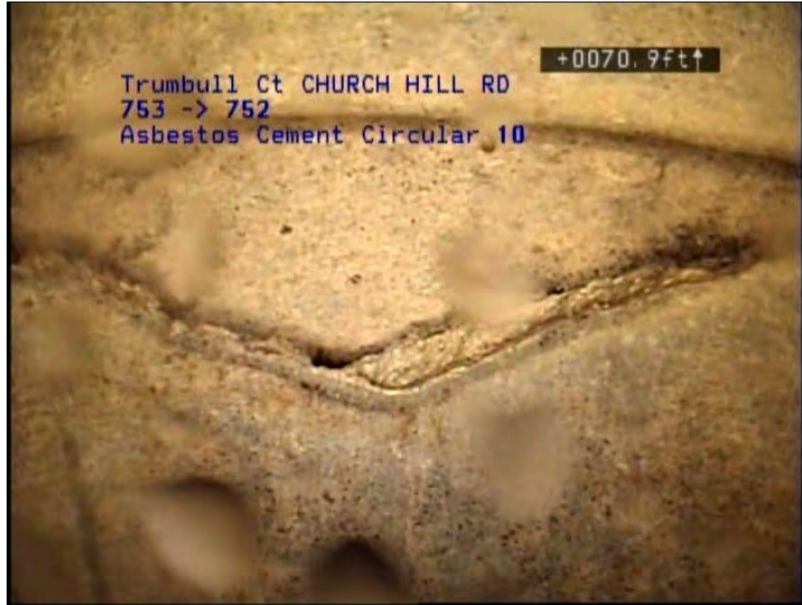
Photo: 378_378_1886_A.jpg, VCR No.: Disc 33 70.9FT, Broken, at 12 o'clock, within 8 inches of joint: YES
