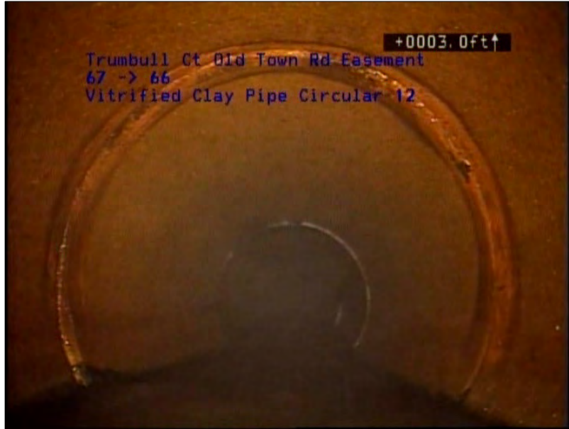
Photo: 535_535_2700_A.jpg, VCR No.: 49 3FT, Infiltration Runner, from 12 to 12 o'clock, within 8 inches of joint: YES
