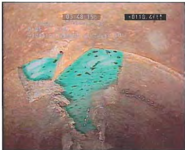
Photo: 118_119_791_A.JPG, VCR No.: Tape #6 118.2FT, Repair Patch, at 12 o'clock, within 8 inches of joint: YES
