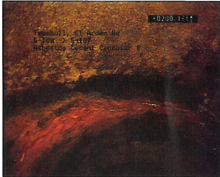
Photo: 31_32_266_A.JPG, VCR No.: Tape 1 280FT, Deposits Attached Encrustation, 5 % of Cross Sectional Area, At 10 o'clock, Within 8 inches of joint: YES
