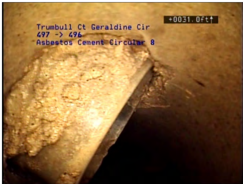
Photo: 213_213_1125_A.jpg, VCR No.: Disc 16 31FT, Survey Abandoned
