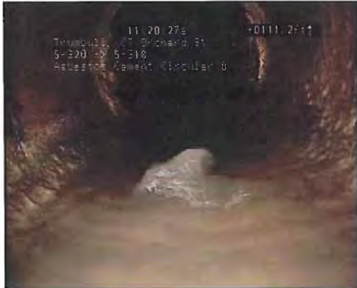
Photo: 79_80_558_A.JPG, VCR No.: Tape #5 111.2FT, Infiltration Gusher, at 06 o'clock, within 8 inches of joint: NO
