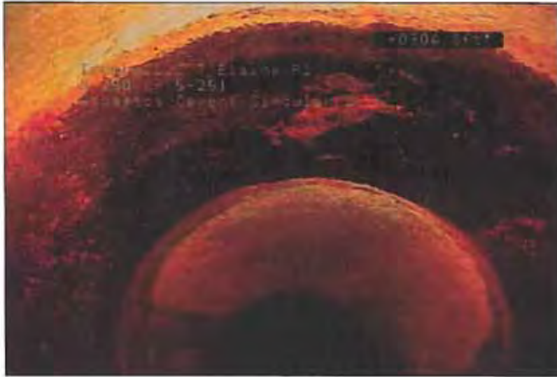
Photo: 118_119_768_A.JPG, VCR No.: disc #13 304.8FT, Deposits Attached Encrustation, 5 % of Cross Sectional Area, From 12 to 12 o'clock, within 8 inches of joint: YES
