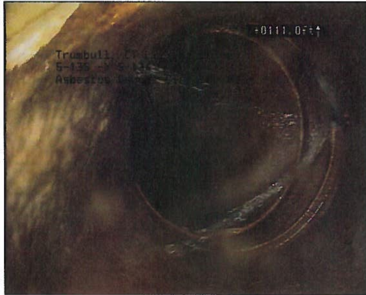
Photo: 17_18_127_A.JPG, VCR No.: Tape 1 111FT, Tap Factory Made Defective, at 10 o'clock, 6", within 8 inches of joint: NO
