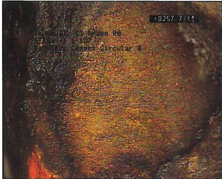
Photo: 31_32_264_A.JPG, VCR No.: Tape 1 257.6FT, Infiltration Dripper, at 10 o'clock, within 8 inches of joint: NO
