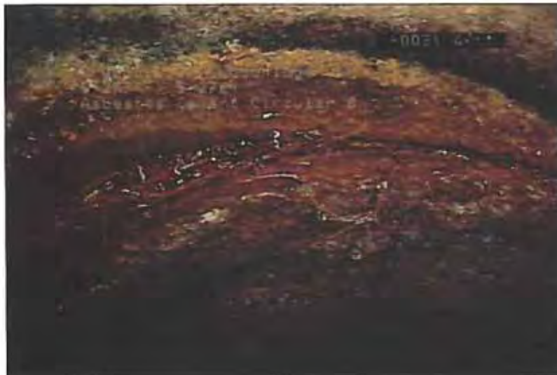
Photo: 84_85_542_A.JPG, VCR No.: disc #10 31.1FT, Infiltration Runner, from 12 to 12 o'clock, within 8 inches of joint: YES
