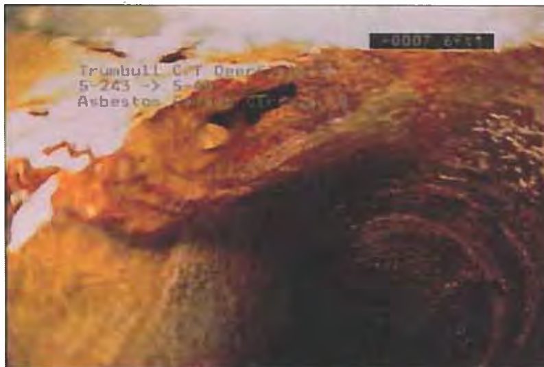
Photo: 114_115_741_A.JPG, VCR No.: disc #13 7.6FT, Infiltration Runner, at 10 o'clock, within 8 inches of joint: NO
