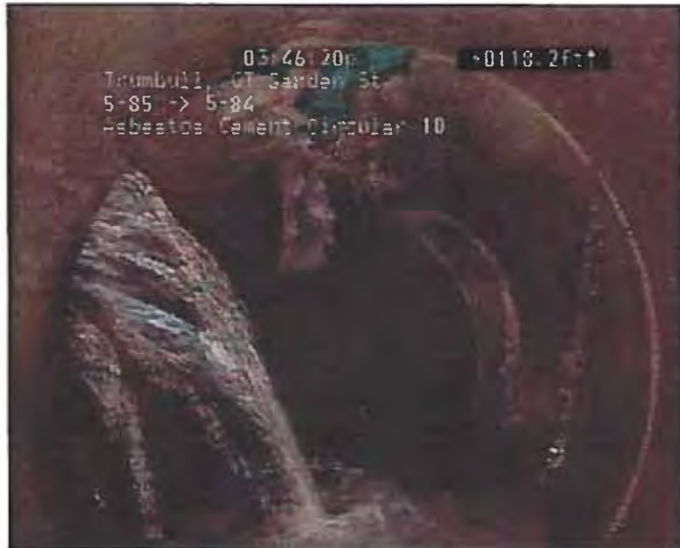
Photo: 118_119_790_A.JPG, VCR No.: Tape #6 118.2FT, Infiltration Gusher, from 08 to 11 o'clock, within 8 inches of joint: YES
