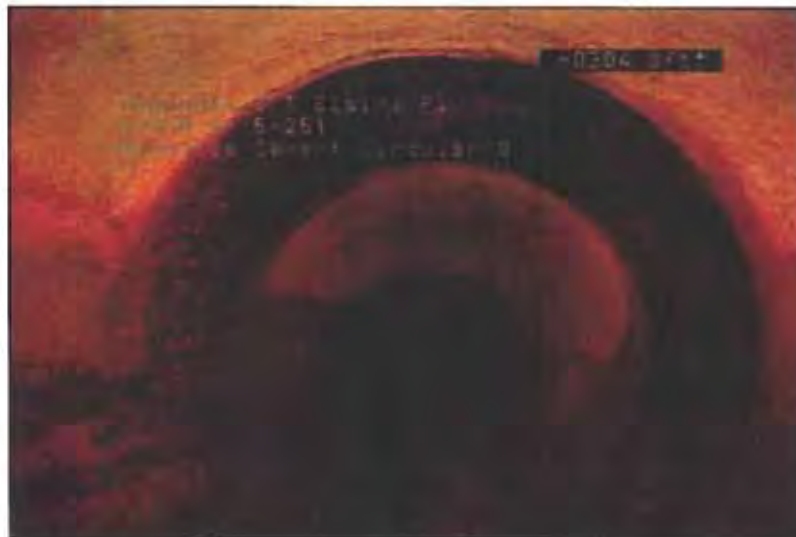
Photo: 118_119_769_A.JPG, VCR No.: disc #13 304.8FT, Infiltration Weeper, from 12 to 12 o'clock, within 8 inches of joint: YES
