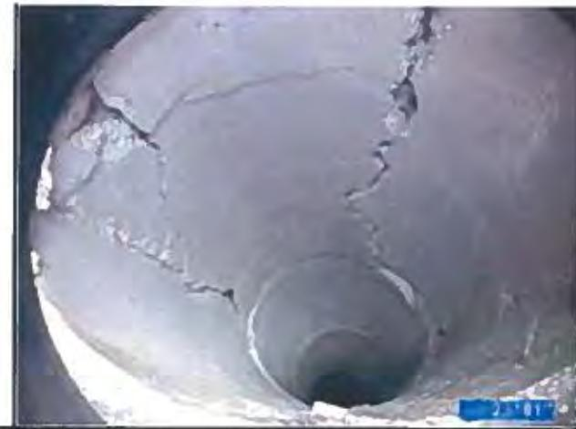
**Conclusion** The pipe is damaged throughout this segment.
