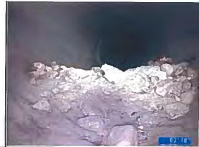
**Conclusion** Significant wear was seen in the pipe bottom, and cracked pipe 57 feet west of DMH S3. Debris stops the camera 84 feet west of DMH S3.
