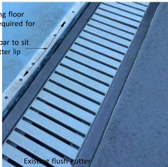
Existing northeast corner, zero entry
