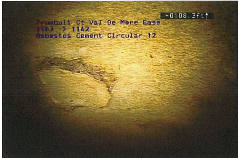
Photo: 172_173_874_A.jpg, VCR No.: Disc # 3 108.3FT, Hole Soil Visible, at 09 o'clock, within 8 inches of joint: NO
