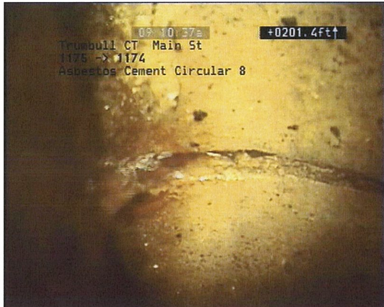
Photo: 49_50_312_A.JPG, VCR No.: 1 201.4FT, Infiltration Runner, at 08 o'clock, within 8 inches of joint: YES
