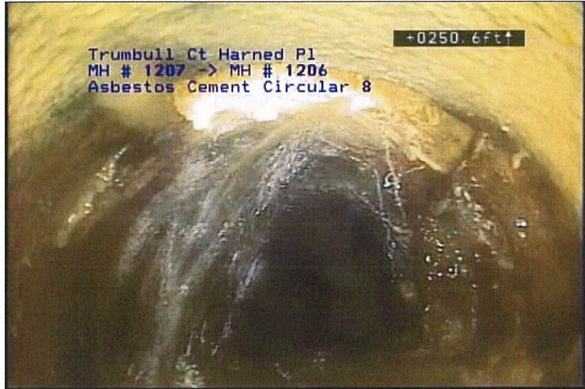
Photo: 45_46_252_A.jpg, VCR No.: Disc # 2 250.8FT, Infiltration Gusher, from 10 to 12 o'clock, within 8 inches of joint: YES
