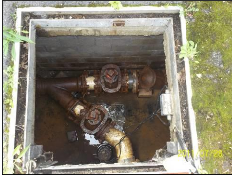
Valve Vault with Emergency By-Pass (By-Pass Connection Shown Below)
