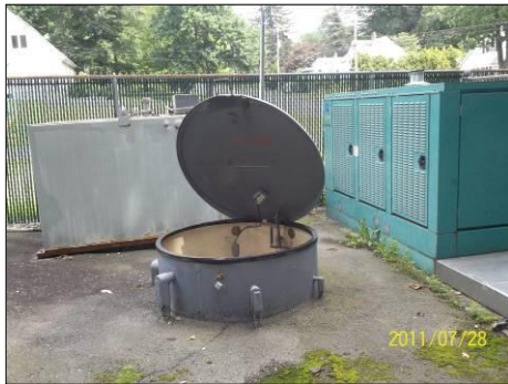
Access Tube to Drywell
